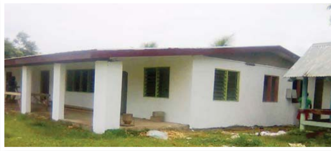
Sabeto Kindergarten nearing completion
